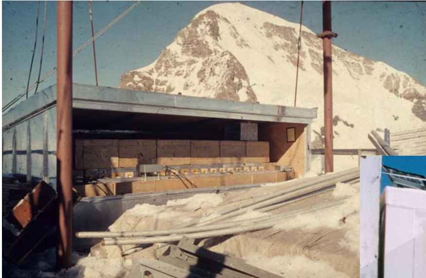
Roof of Sphinx building
